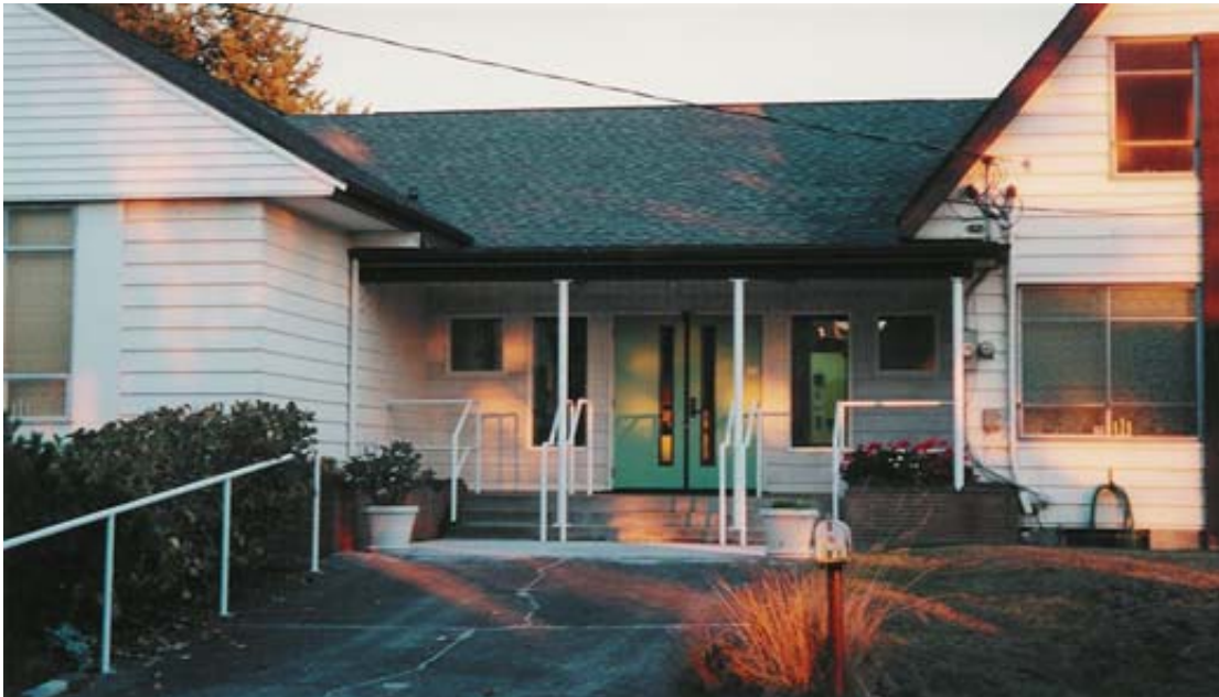
After — Exterior of main entrance. Four new windows, windows in two doors, improved finishes, and a new handrail at the entry ramp help project a more welcoming appearance to the street.
