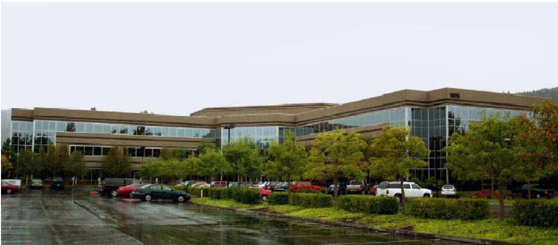
Exterior of Building
