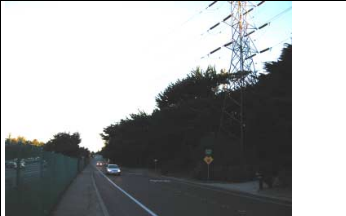
Base of pole is within 20 ft of residence. Note location of “stop sign ahead” post relative to street and HWY 280.
