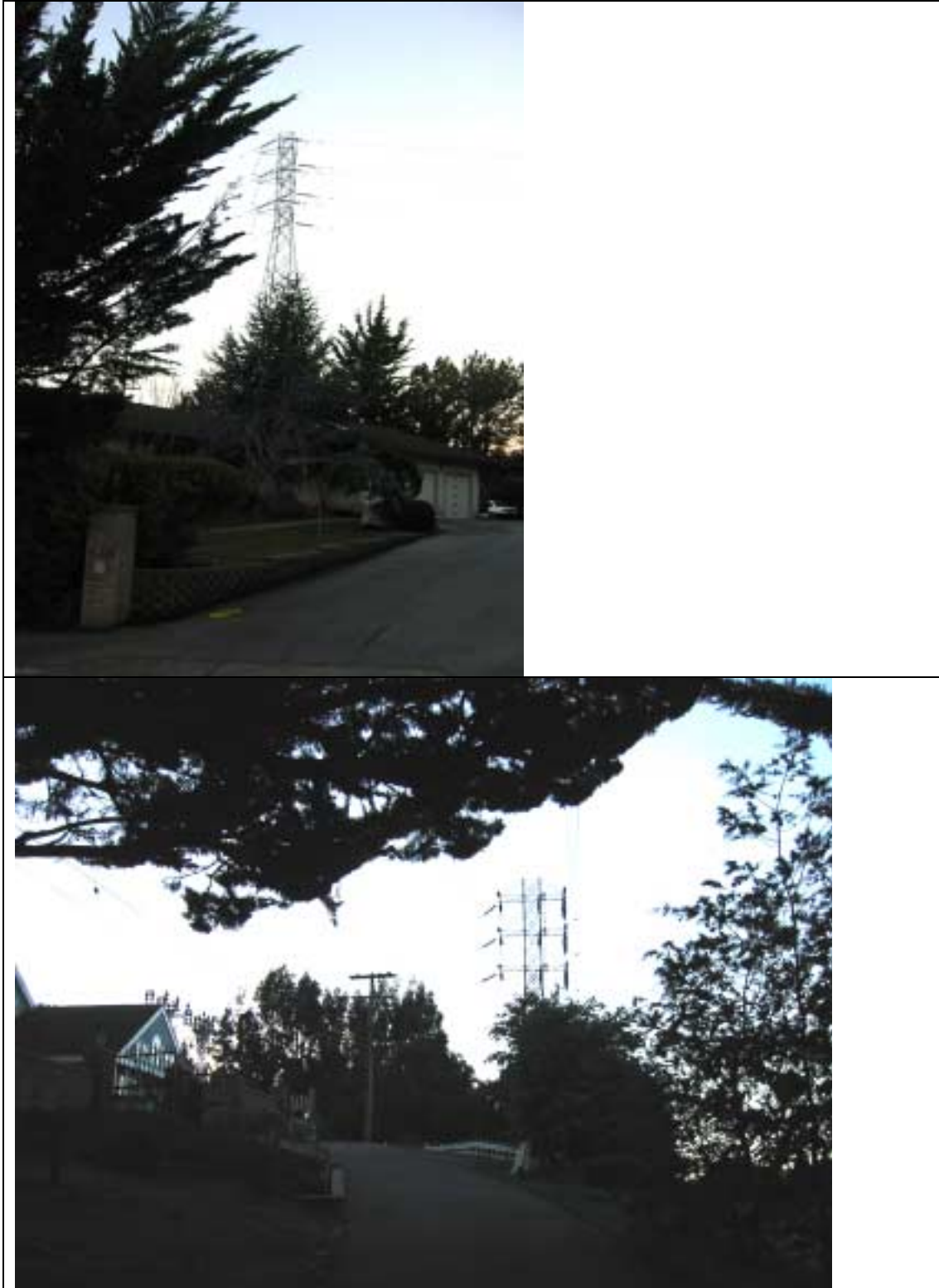
In many instances 100 ft rights of way overlap private residences. Existing towers are within 20-50 ft of residences.
