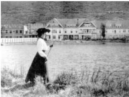
A woman wears a "classic period" hat in this photo that depicts the Hot Lake Sanatorium in 1906 during the construction of its brick addition. - Photo from "The Hot Lake Story," obtained courtesy of Fred Hill
