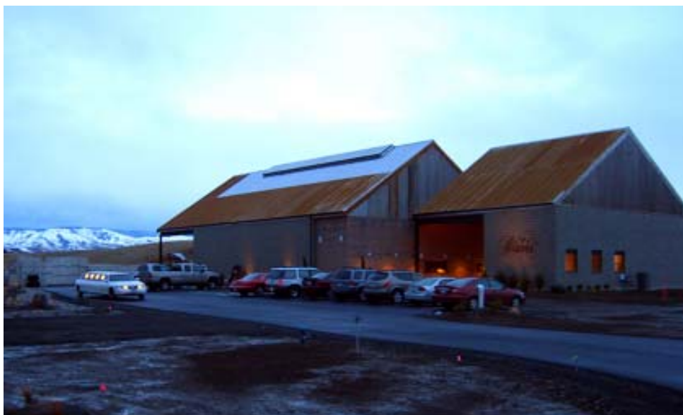
Waters new facility south of town
