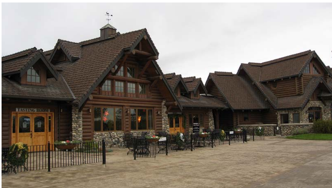
Entranceway to Basel Cellars
