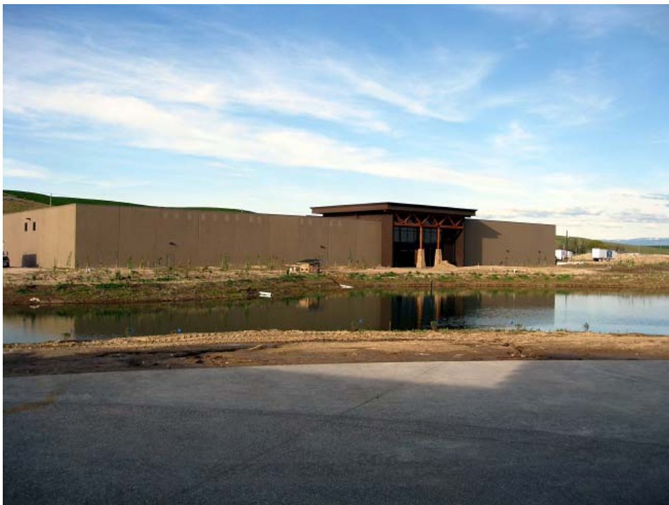
Precept's new production facility on the way in to Walla Walla
